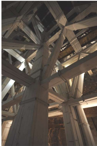
Fig 1. Wooden truss-type support in an excavation mined by block working- Michałowski cavern, salt mine Wieliczka (author: ACM).
